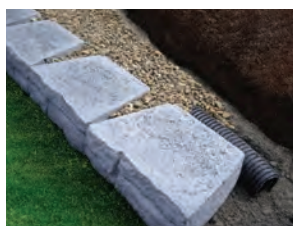
5. Lay drain coil and drainage aggregate
