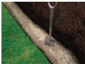
1. Mark out and dig trench
